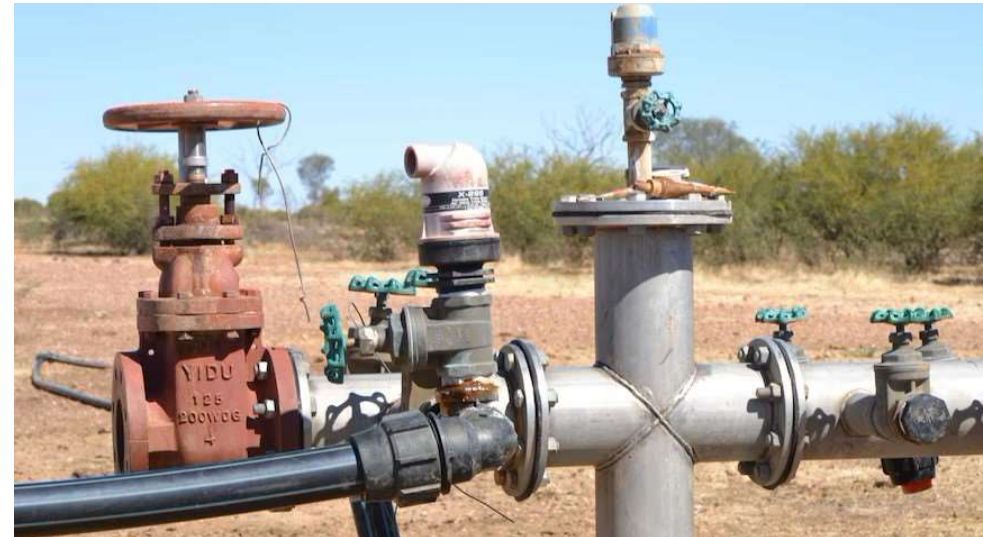
Source : A capped bore in western Queensland, funded through the Great Artesian Basin Sustainability Initiative, Virginia Tapp
